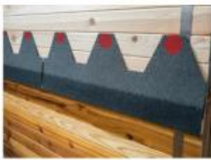
fasten the shingles with screws
